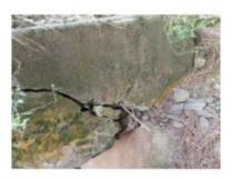
Figure 4 Superstructure pathologies: torsion cracks, steel corrosion, shear crack at Abutment B
