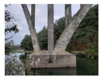
Figure 3 Substructure pathologies: concrete cracking, vegetation, concrete efflorescence
